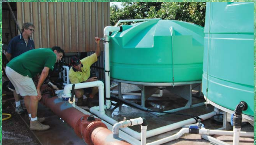
Laurie takes Les and Peter through the workings of his automated fertigation system.
