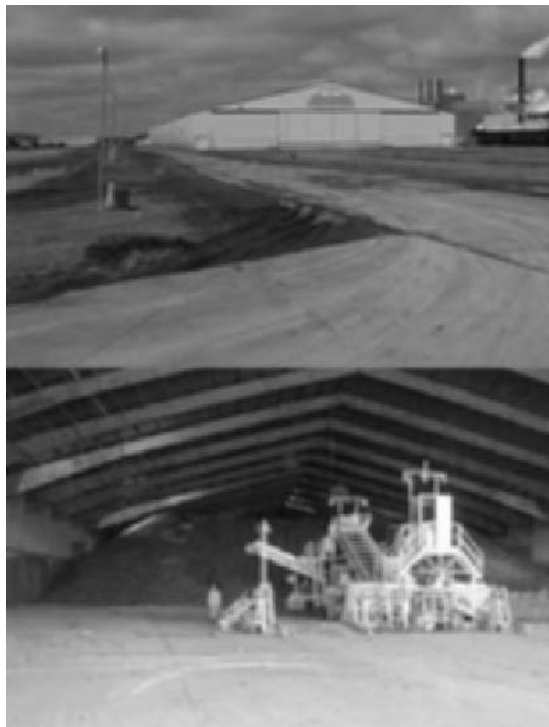
Fig. 15.7 Interior and exterior views of sheds used to store frozen roots for processing late in the campaign (American Crystal Sugar Co.).
