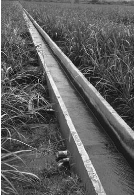
Fig. 5.8 Drop spile canal system in Swaziland.
