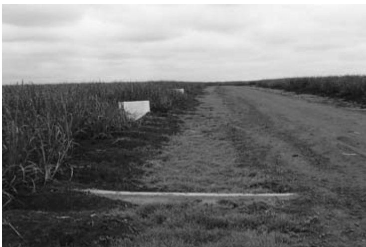
Fig. 5.17 Grass lined tail drain with wide and shallow profile.
